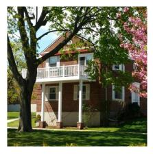
Steel or Wood posts are permitted. GOVO recommends that steel posts be used. Steel posts will cost approximately \$2,000 more than wood but will require significantly less maintenance in the long run than wood.
