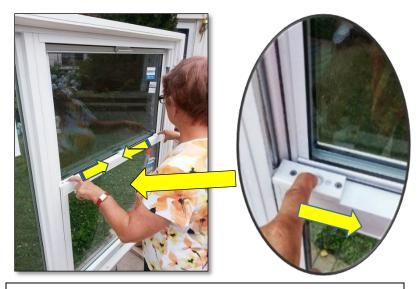
**2.** PUSH BOTH TABS ON TOP OF WINDOW SASH AT SAME TIME TOWARDS THR MIDDLE TO UNLOCK WINDOW.
